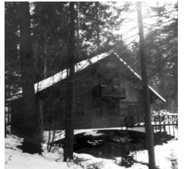
1938 - Bridge with a mountain lodge on top of it. Sketches and photographs preserved in the Pizzigoni archive at the Public Library of Bergamo. The wood cladding was extended further down in a later stage and at the moment also the span of the bridge is filled in to become a kind of basement space.
